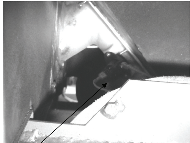
Manual reset 225 deg. Normally closed high temp disc
