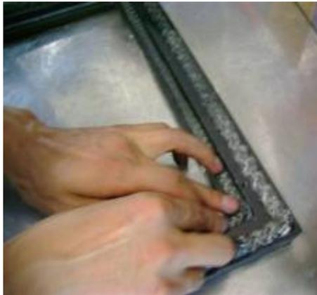
3. Place glass on top of the inner gasket. Make sure glass is centered in the opening top to bottom and left to right.
