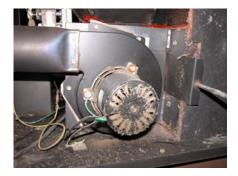
This is a picture of an exhaust blower that was not maintained correctly, which caused the stove to run in-effectively. This blower was replaced.
