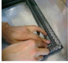
3. Place glass on top of the inner gasket. Make sure glass is centered in the opening top to bottom and left to right.
