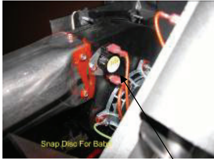
Proof of Fire 110 °Low Limit Safety Sensor, Normally Open
